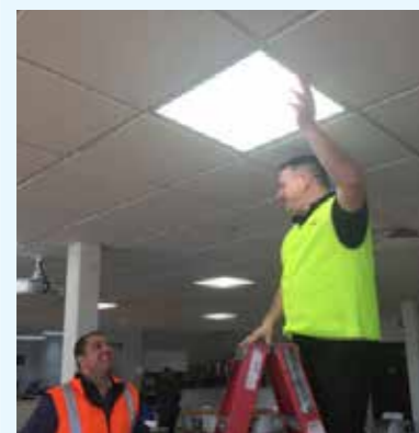
Engineering Manager at Aspen's Dandenong site inspecting the newly installed LED light
