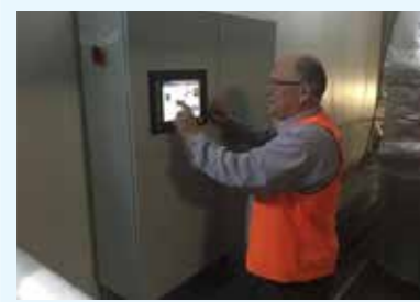
Facilities Manager of Aspen Dandenong operating the new Supervisory Control and Data Acquisition (SCADA) system
